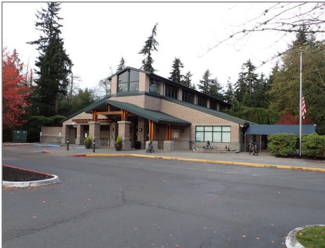
Mukilteo Library during the morning of the follow-up site visit.
