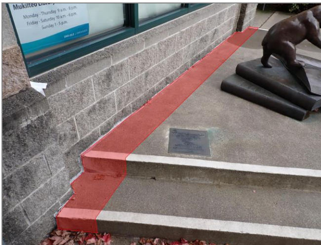
Proposed poured slab removal section.
